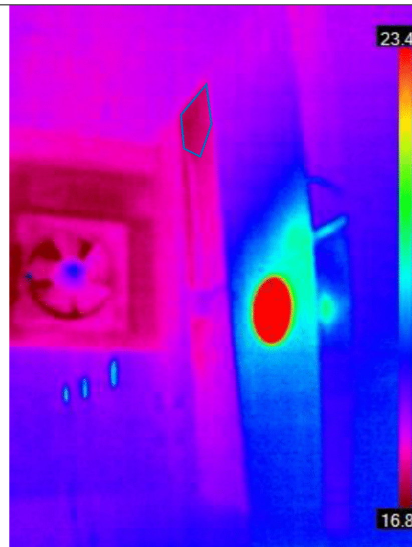
Ceiling of kitchen
